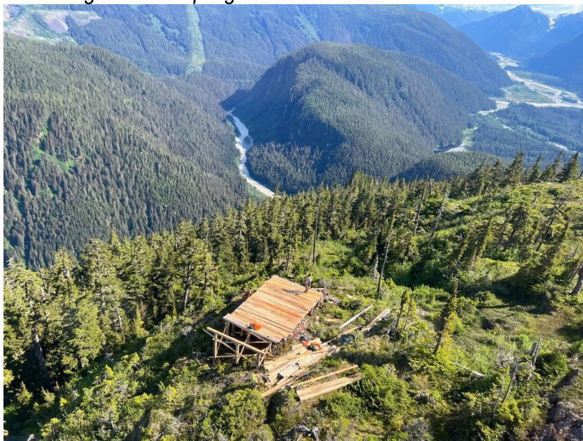
Photo 1: Drill pad under construction
